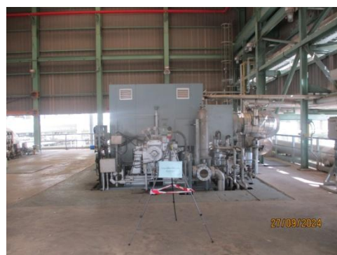
Propylene Compressor (R-650)
